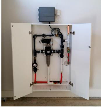
Most IrriGRAY installations in new homes have the filter / water management module and controller installed in the garage.
